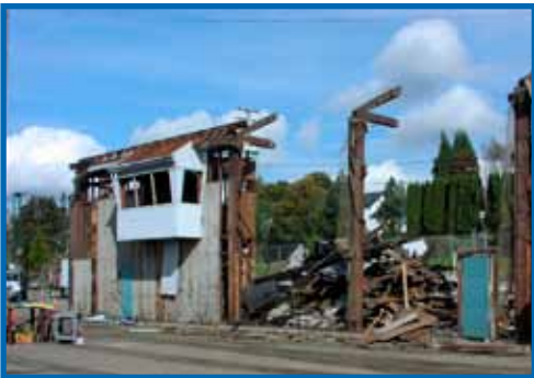
What was known as building #1 and the drying kilns being demolished.
