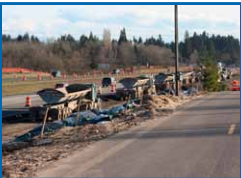
Trucks lineup south of the new interchange waiting for fill.
